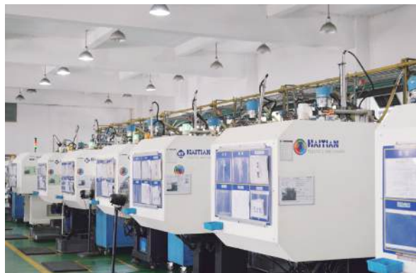
集中供料系统 Centralized feeding system
